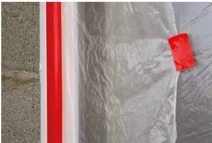
Use a straight edge for a clean and straight line in masking applications
